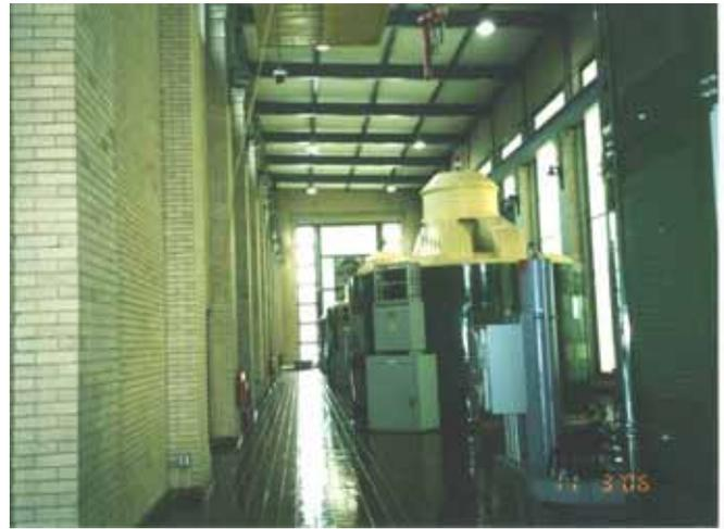
*A view down the generator hall. The hydroelectric turbines are located underneath each generator, about 20 feet below the floor.*
